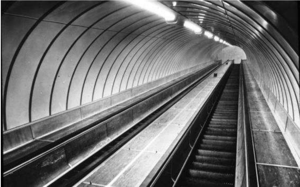
Figure 41 Archival imagery of Tyne Pedestrian and Cyclist Tunnel
